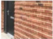
2: Example of protruding brick banding entrance areas.
